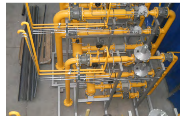
Visoko for the company BH GAS Ltd. (Bosnia and Herzegovina) MAIN REGULATION - MEASURING STATION Q = 30.000 \text{ m}^3/\text{h} | p = 50 \text{ bar}
