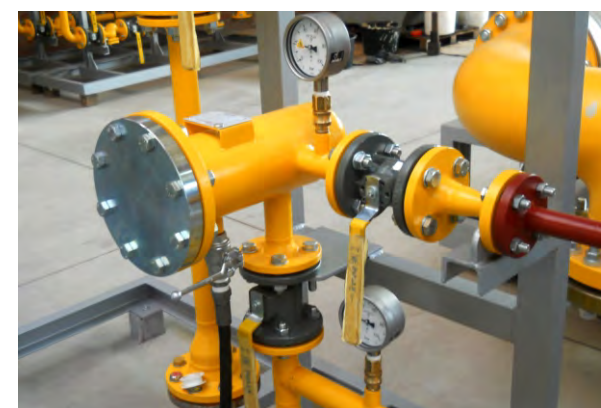
Gas filter DN125 PN16 (Angle installation)
