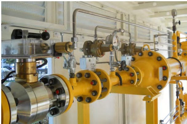
Place of installation: SBK for the company BH GAS Ltd. (Bosnia and Herzegovina) MAIN REGULATION - MEASURING STATIONS Q = 6.500; 10.000; 20.000 \text{ m}^3/\text{h} | p = 19 - 50 \text{ bar}
