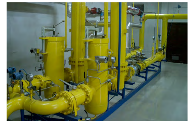
Visoko for the company BH GAS Ltd. (Bosnia and Herzegovina) MAIN REGULATION - MEASURING STATION Q = 30.000 \text{ m}^3/\text{h} | p = 50 \text{ bar}
