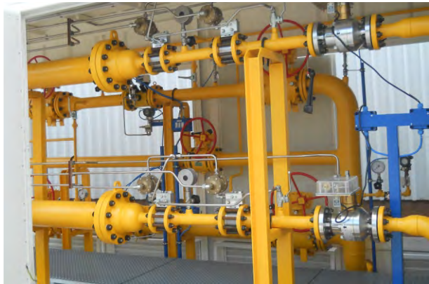
Place of installation: SBK for the company BH GAS Ltd. (Bosnia and Herzegovina) MAIN REGULATION - MEASURING STATIONS Q = 6.500; 10.000; 20.000 \text{ m}^3/\text{h} | p = 19 - 50 \text{ bar}
