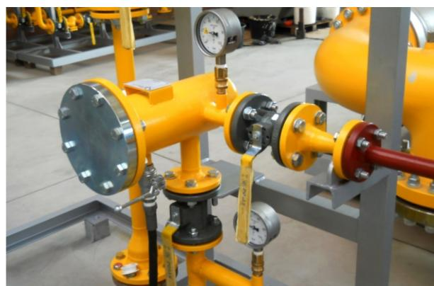
Gasni filter DN125 PN16 (Ugaona ugradnja)
